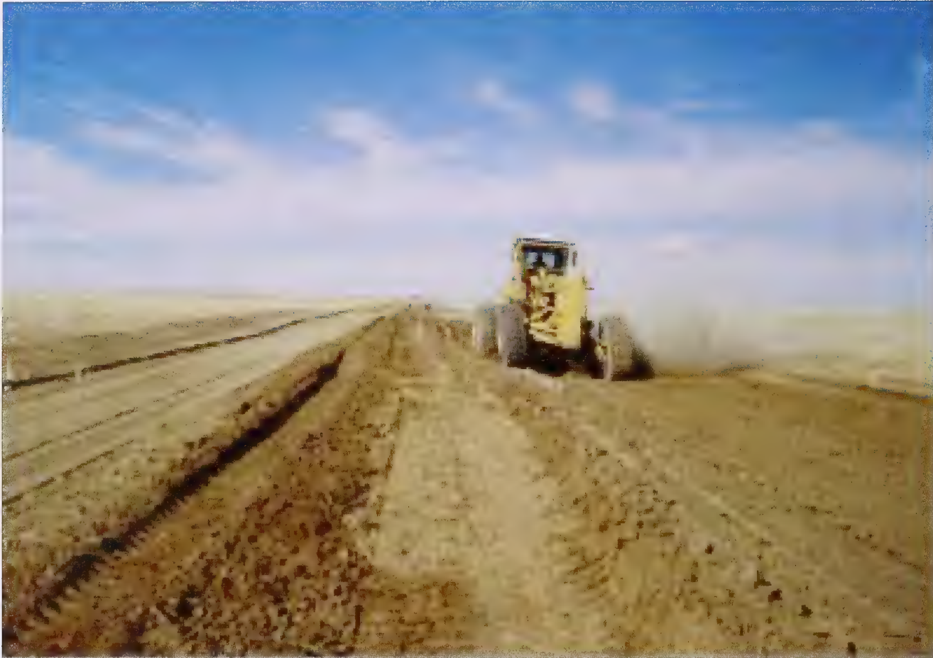
Photo 28 Double blade width stripping
